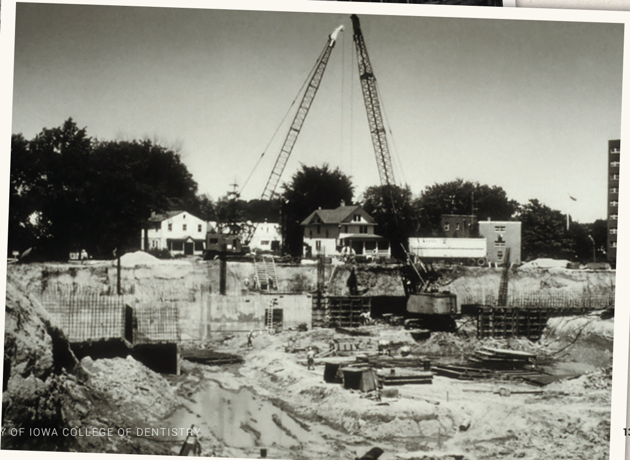
Original foundation construction of the Dental Sciences Building, 1973.
